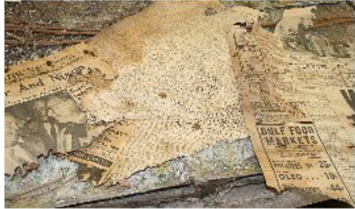
Newspapers were used to insulate the floor and were placed directly on top of the wood floor boards.
