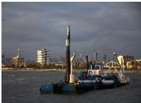
Dredging sand for the beach
