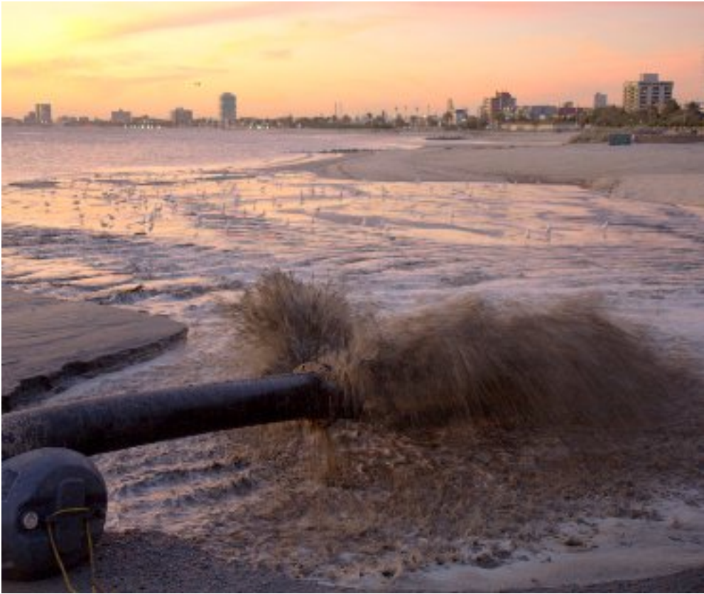
Sand dredging to build up the beach
